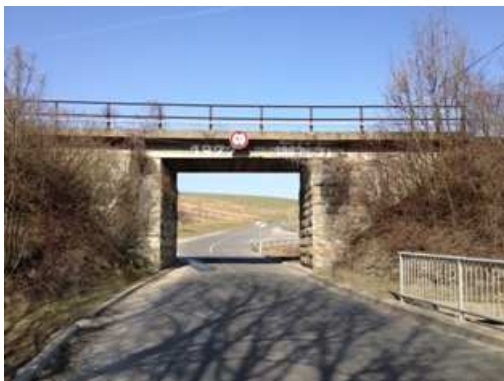
Obr. 23 viadukt v Bojkovicích (Bor, 03/2013)
