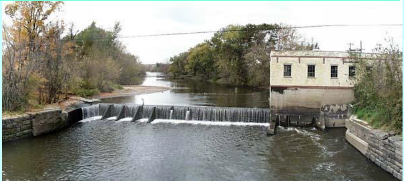
Linen Mill Dam, Baraboo River (above). Removed October, 2001 (below).
