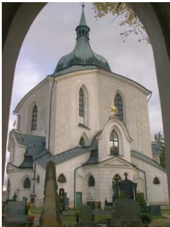
The pilgrimage church of St. John of Nepomuk in Zelená hora near Žďár nad Sázavou. (Photo: archive)
